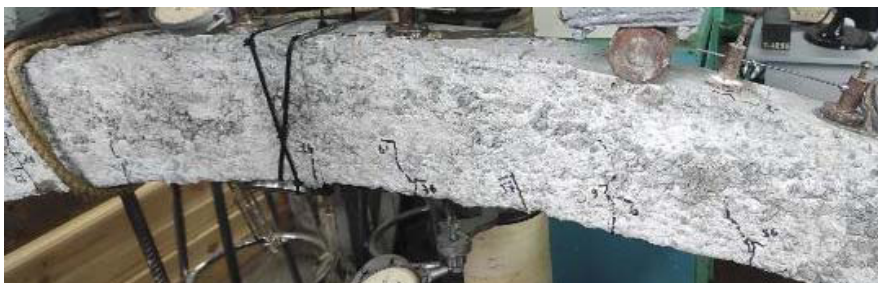
Figure 7. General view of the A2 arch after testing
